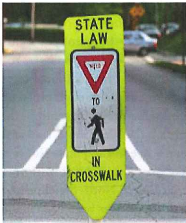
In-roadway warning sign.
